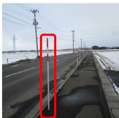
Installed poles to prevent collision course phenomenon
